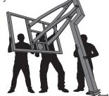
**Step 7:** Fasten pole to threaded ground anchor plate by installing and hand tightening the three rear anchor bolts with lock washers.
